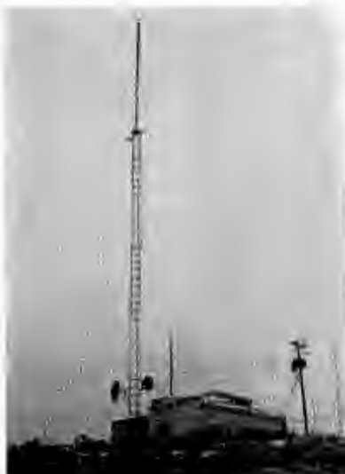
Radome-covered microwave dishes are mounted on the TV tower at both transmitter sites. Shown here is the KNDO-TV transmitter building at Ahtanum Ridge.
